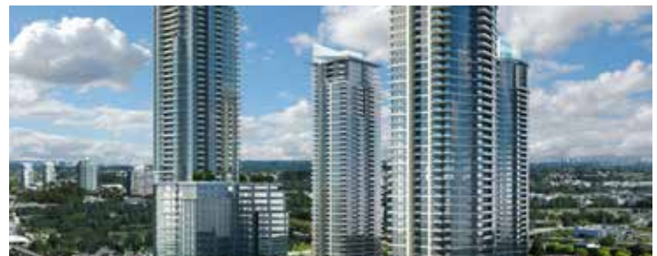
Solo District will deliver an additional 230,000 sf of office space as part of the project’s second phase scheduled for completion in late 2015.
