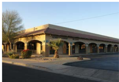
Southern Business Center 777 W. Southern Avenue, Mesa, AZ 85210
