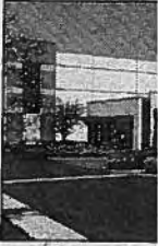
Largest new industrial construction in N
