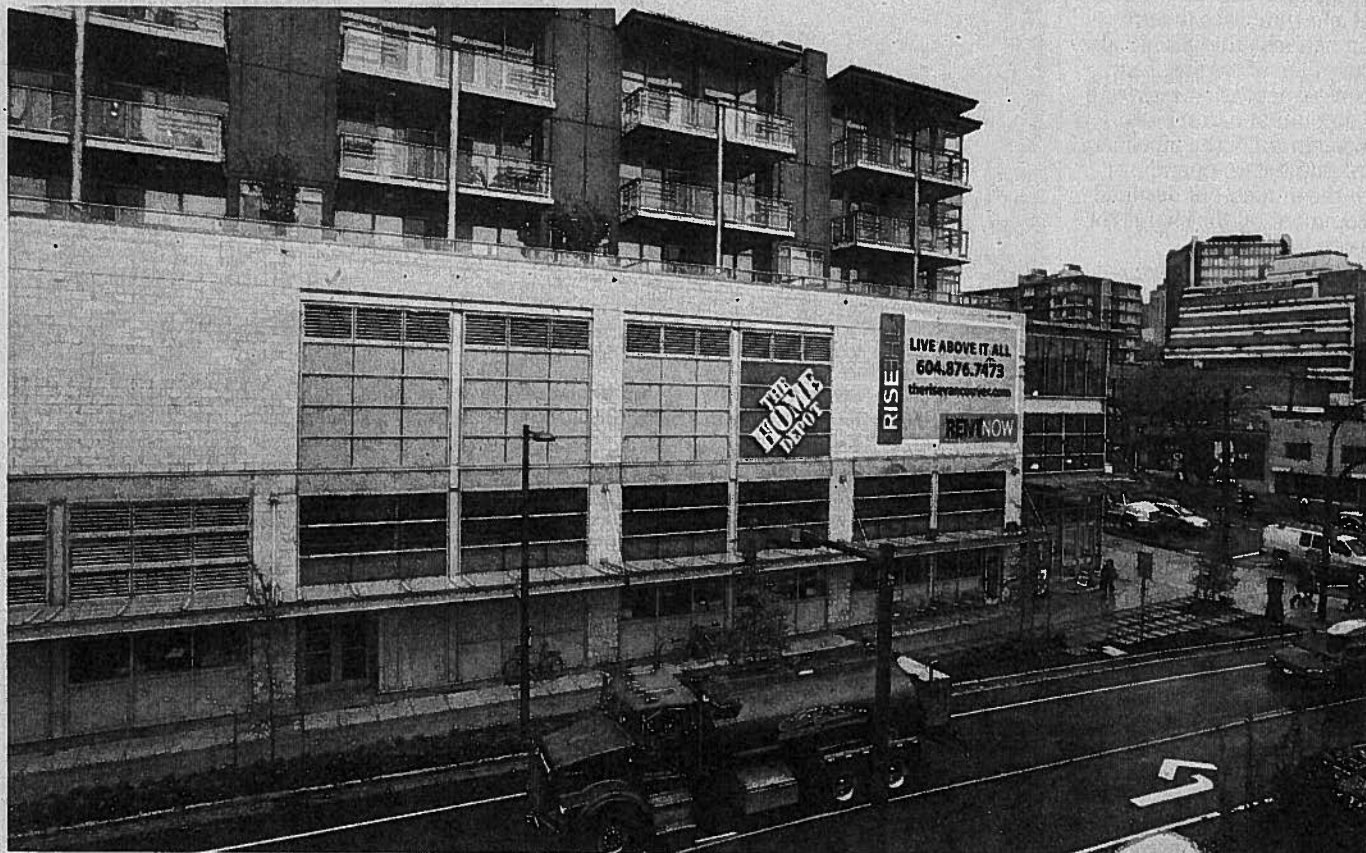
Designers of the Rise, a mixed-use development in Vancouver, had to come up with an underground loading area so residents wouldn't be annoyed by deliveries or garbage pickup. LAURA LEYSHON FOR THE GLOBE AND MAIL
