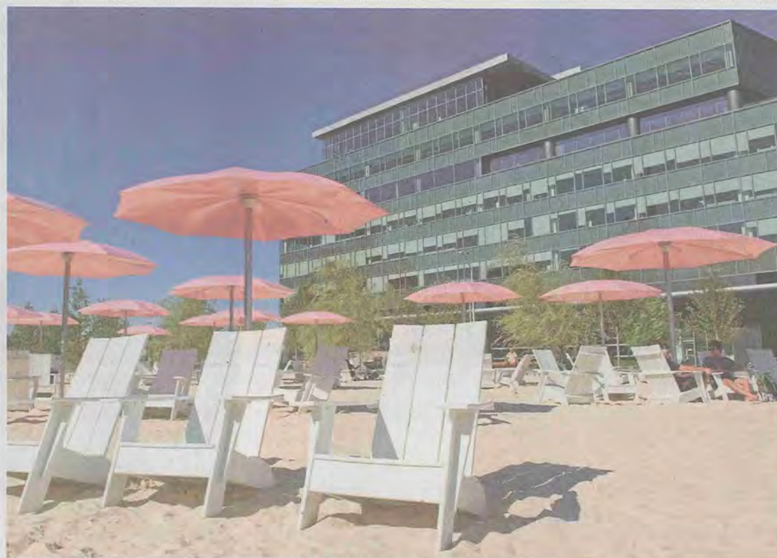
The lively new headquarters of Corus Entertainment lies next to Sugar Beach on Toronto's waterfront. Below, the city's new Telus House aims to make a green impression. SARAH DEA/THE GLOBE AND MAIL
