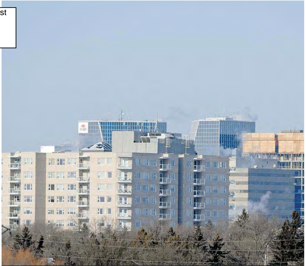
The crane works on Hill Centre Tower III on Thursday. Regina is the tightest major office market in Canada, a title the Queen City looks unlikely to concede any time soon. Photograph by: Troy Fleece, Leader-Post, Leader-Post
