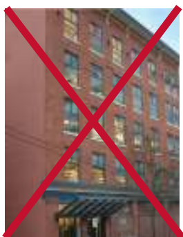
840 Cambie Street Converting to residential
