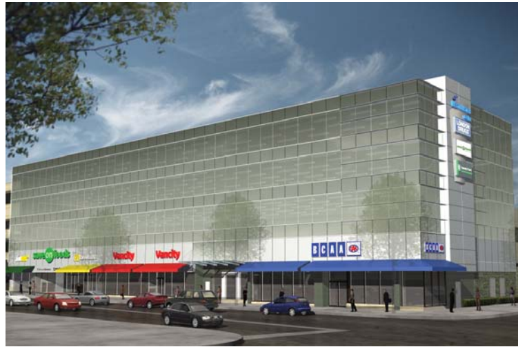
UPG Group's 42,000-sf addition to Westminster Centre South Office Tower (505 6th Street) will come on stream in fall 2008
