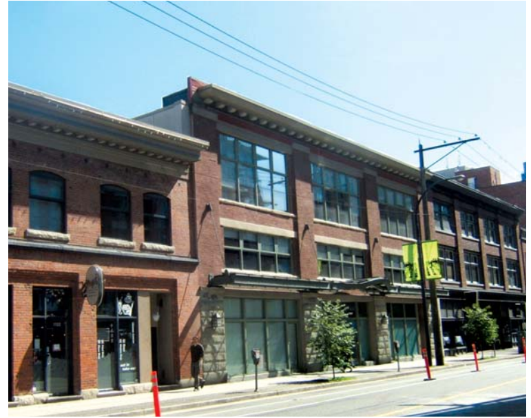
1128 Homer currently offers the only large block of available space in the Yaletown marketplace
