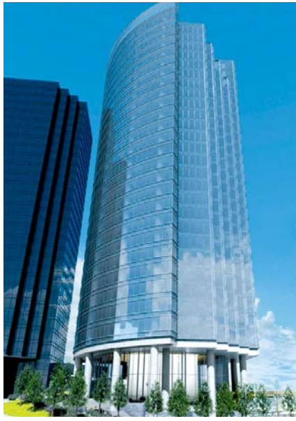
The shovels are poised to break ground at Ivanhoe Cambridge's 398,607- sf Metrotower III
