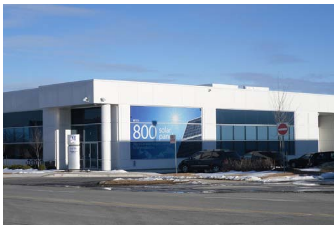
The LoyaltyOne call centre at 6696 Financial Drive in Mississauga features the largest rooftop solar panel installation in Canada.
