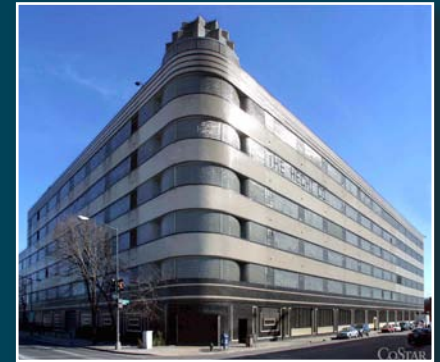
The six-storey, 550,000-sf building known as "Building A" in Patriot Yards is the largest block of available industrial space in the Washington market today. The recognizable art deco-styled building was built in 1937, and served as Hecht's distribution center until 2007. Patriot Yards is sited prominently on New York Avenue, the gateway to Washington, DC from the east.
