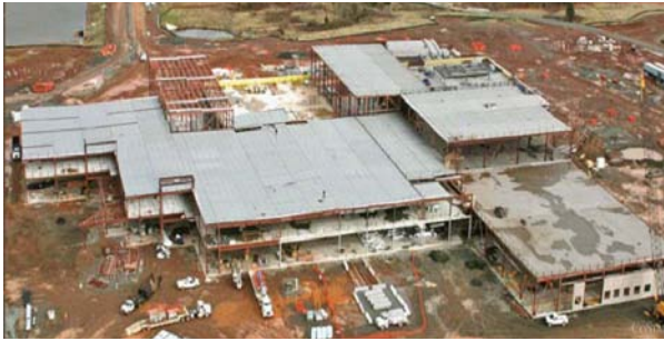
Covance purchased this partially constructed building from Eli Lilly.
