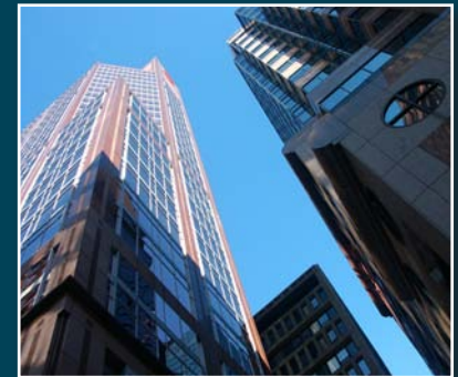
Downtown Montreal office towers
