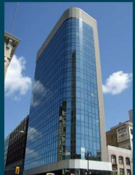
275 Portage Avenue, Kensington Building
