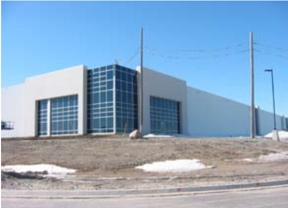
6200 Millcreek Drive, Mississauga
