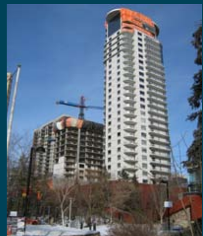
The Icon Towers I & II, provided by Langham Properties Ltd.
