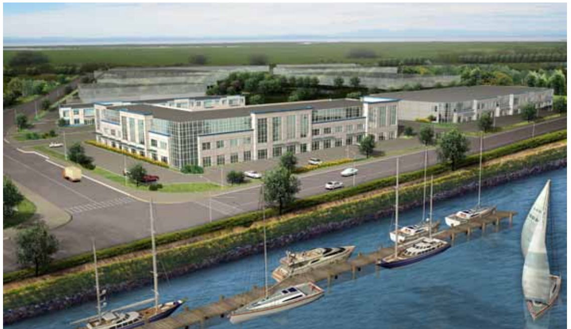
Phase II of Farrell Estates Ltd.'s Shelter Island project will be complete June 2010. The next phase is in the planning stages.
