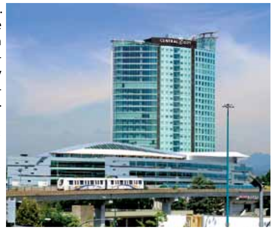
Simon Fraser University will expand by 16,000 sf at Central City (13450 102nd Avenue) in 2010 when the university trades two floors for 50,000 sf on the podium level
