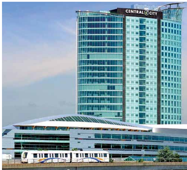
Office space recently made available at Central City in Surrey is fully leased
