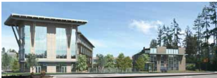
Citimark and Darwin Construction plan to break ground by year-end 2010 on Building C at Dollarton Business Park .
