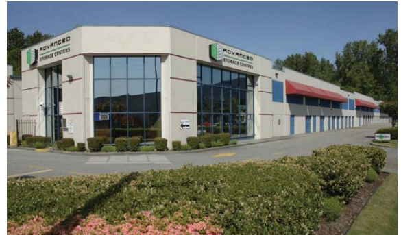
A property in the ACM portfolio of self-storage facilities that sold in 2004 for $35,700,000. Avison Young represented the buyer.
