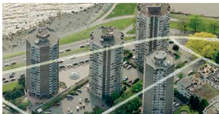
The sale of the four-building, 598-unit Beach Towers in Vancouver's West End in December 2009 for $117 million was BC's second largest multi-family sale in 2009. The largest was Langara Gardens (West 57th and Cambie, Vancouver) for $157 million.
