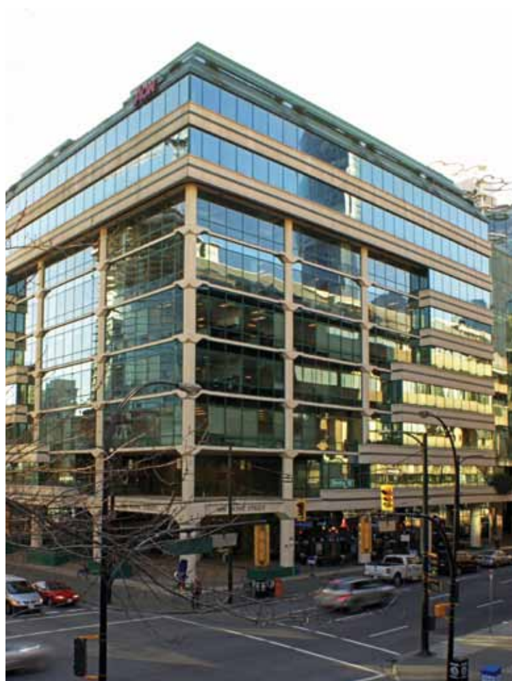
GWL Realty Advisors' sale of 900 Howe to a private buyer in December 2009 represented the only sale of a class A building downtown in the fourth quarter of 2009. The 103,000-sf building is 100% leased.
