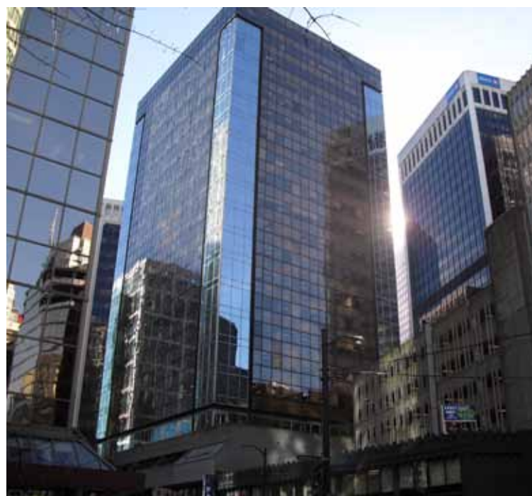
1050 West Pender Street (above) and 1090 West Pender Street were part of an ownership swap with an eye to future redevelopment potential
