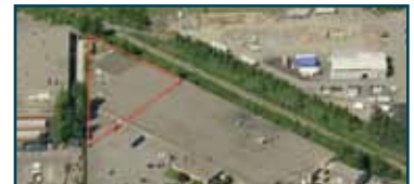
12179 86 AVENUE, SURREY • Up to 27,950 sf • Cost-effective warehouse space • 2 dock loading/3 grade loading doors • Heavy power Contact: Jot Mattu
