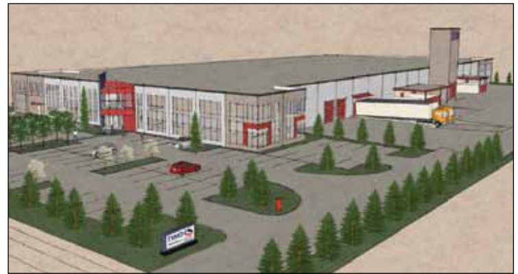
Avison Young acted for the user, TWG , in the design-build of a new $14-million facility in Surrey. The 110,000-sf manufacturing warehouse is slated for completion in spring 2011.
