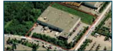
26835 GLOUCESTER WAY, LANGLEY • Freestanding building • 59,259 sf total • 5,125 sf office • ESFR sprinklers and heavy power • $.595/ sf in year one Contact: Michael Farrell / John Eakin
