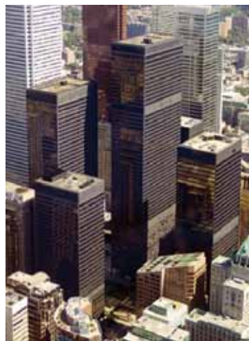
TD Centre Complex
