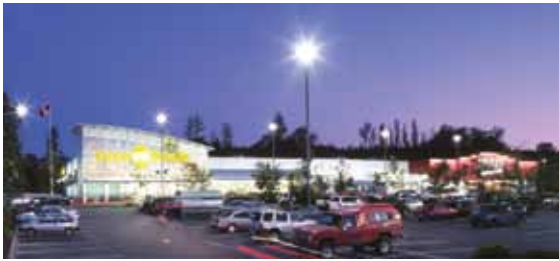
Grosvenor Americas sold South Point Exchange shopping centre in Surrey, BC to a Canadian private investor for $91 million in August 2010. Avison Young acted on behalf of the buyer.
