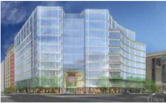
2200 Pennsylvania Avenue NW is a 432,900-sf class A office building being developed by Boston Properties in Washington's CBD. Delivering in February 2011, the building was substantially preleased to law firm Hunton & Williams .
