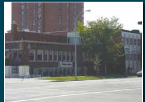
The retail/office building located at 444 5 Avenue South was purchased by a local buyer in spring 2010.
