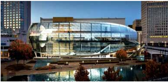
Ottawa's newly redeveloped Ottawa Convention Centre is taking shape.
