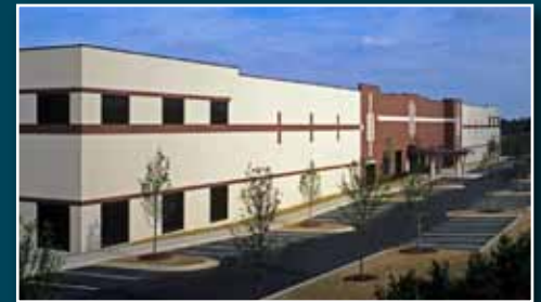
7780 Spence Road is a 798,296-sf class A industrial warehouse building located in Fairburn, GA
