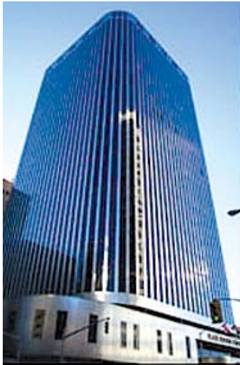
Export Development Corp. (EDC) plans to relocate from 234 Laurier (above) to Canderel Developments' new 450,000-sq.-ft. head office, at the corner of O'Connor and Slater in 2011
