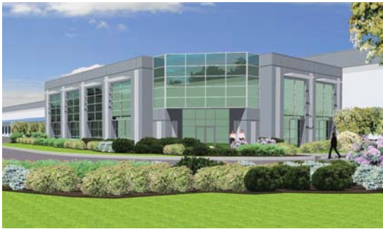
Avison Young recently represented Brewers Distributor Ltd. in the 451,047-sq.-ft. build-to-suit expansion and relocation of its Lower Mainland distribution warehouse to Port Coquitlam, B.C.
