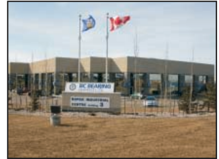
Roper Industrial Centre 59 Street & Roper Road, Edmonton
