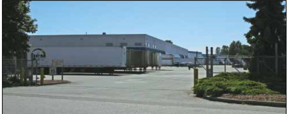
Dayhu Investments Ltd. acquired this warehouse and distribution facility at 450 Derwent Place in Richmond from Rimrock Investment Corporation for $16.5 million. It is the second-largest Metro Vancouver industrial property sale to date in 2010.
