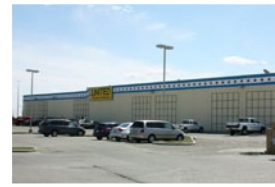
3451 Sunridge Way NE 29,000 sf Northeast Industrial Sublease Opportunity
