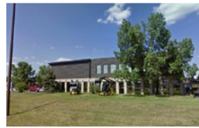
3611 - 60th Avenue SE 15,725 sf Southeast Industrial Leasing Opportunity
