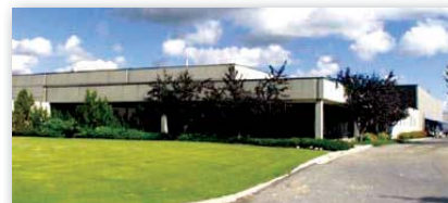
HIBBERT BUILDING • $5,540,000 3202-12TH AVENUE NE • 53,700 sf CALGARY, AB
