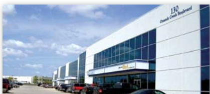
130 OMANDS CREEK • $10,000,000 BOULEVARD • 113,000 sf WINNIPEG, MB
