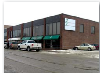
CITY OF RED DEER OFFICE BUILDING • $2,300,000 4815-48TH STREET • 14,500 sf RED DEER, AB
