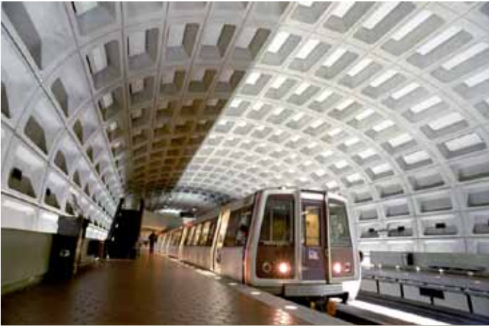
A Washington Metropolitan Area Metrorail System (Metro) underground station.
