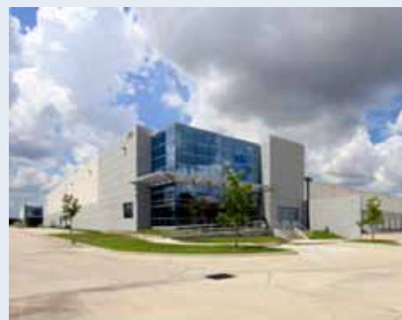
Avison Young represented K2 Logistics in securing a new 142,743-sf distribution facility for the relocation and expansion of K2’s Houston operations.
