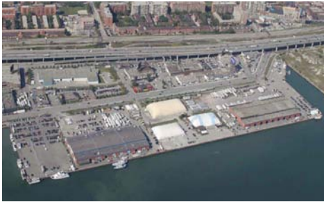
Toronto's East Bayfront District - Existing. Source: WATERFRONToronto
