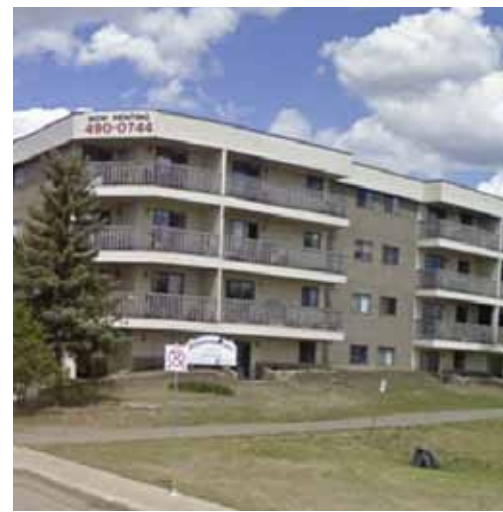
Ridgewood Court (2303 - 38 th Street) is a 94 suite property acquired by Har-Par Investments in 2011 for $9,050,000.
