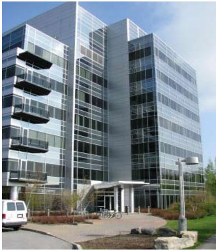
Best Building, 411 Legget Drive, Ottawa
