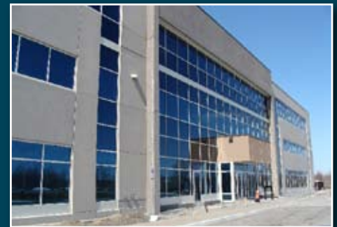
Dell Building, 1001 Farrar Road, Kanata
