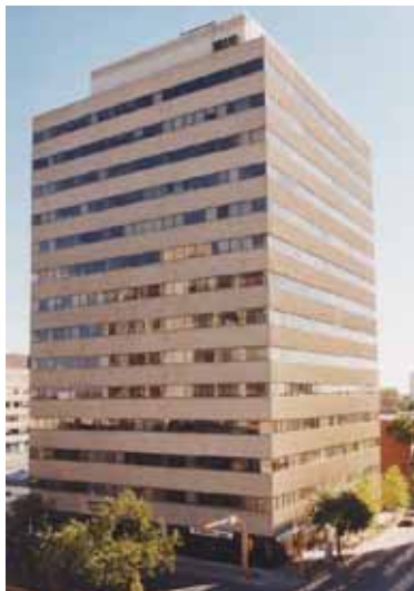
Victoria Tower 145,000 sq.ft. office investment property sold in 2004. The seller was represented by Avison Young.
