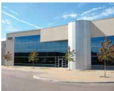
Avison Young represented an international cosmetics company in leasing approximately 200,000 square feet of Industrial space at 550 Petrolia for their new distribution centre.
