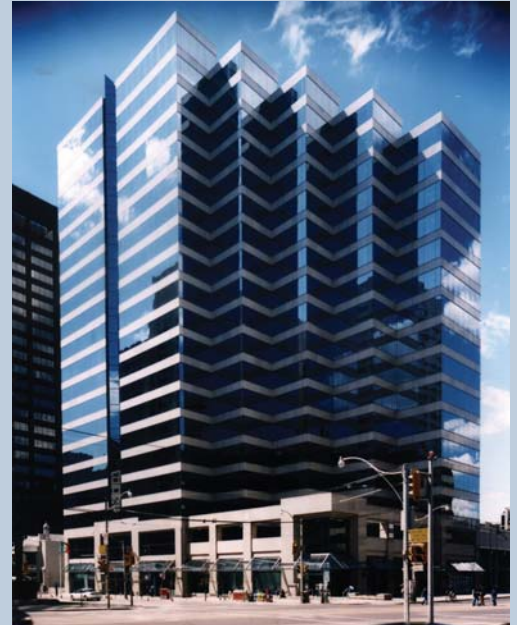
First Century Tower, 438 University Avenue
