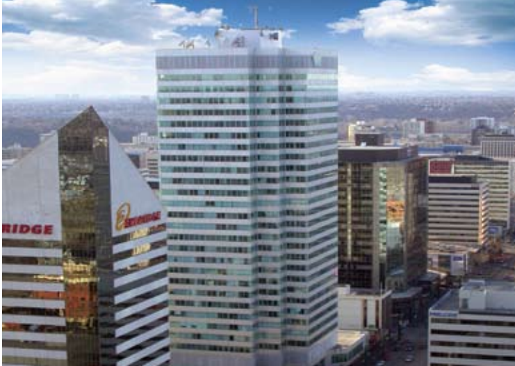
Canadian Western Bank Place is a class A building located in the financial district.
